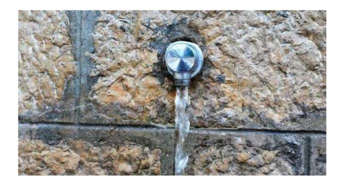
Turn off all exterior faucets and drain water from outdoor pipes, valves and sprinkler heads to prevent pipe bursts.
