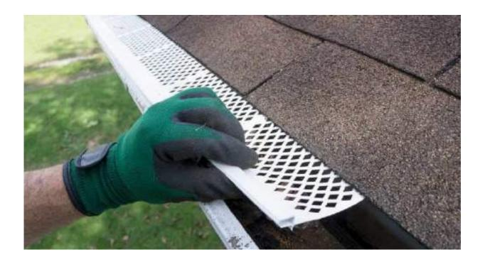
Clean gutters allow water to easily flow down from your rooftops and away from your home, preventing damage to your foundation and ice buildup on your roof.
