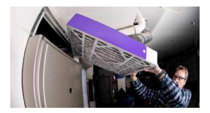
Replace the furnace filter monthly to ensure efficiency and keep dust particles from penetrating the clean, heated air. Inspect your furnace for leaks and test for carbon monoxide.
