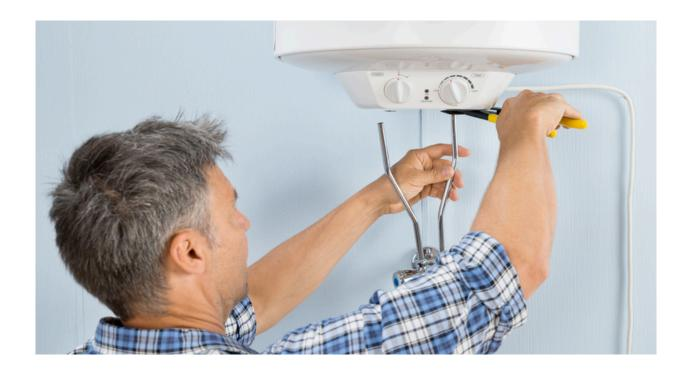
Particles and sediment can collect over time in the bottom of your water heater, hindering the unit's efficiency.
