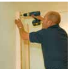
1. SWIP Studs fixed to wall
