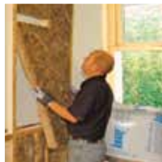
2. SWIP Batt between SWIP Studs
