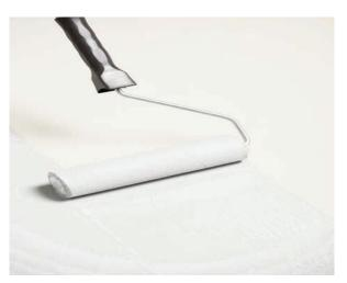
The quantity of material used per coat and the number of coats may vary dependant on the porosity of the substrate and the surface profile. If a slip resistant profile is required, the first coat is completely blinded with **SpECtop NS GRAINS**. This should be carried out while the coating is still wet.
