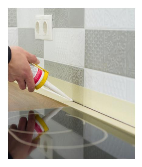
Whether you have grout or caulk as a filler between your tiles in the bathroom, it will exhibit signs of wear and tear over time. If you notice any crumbling, peeling, or mildew, it's probably time for a touch-up.
