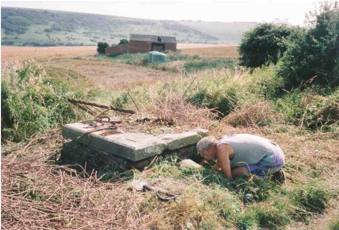
Renovating Harvey's Cross
