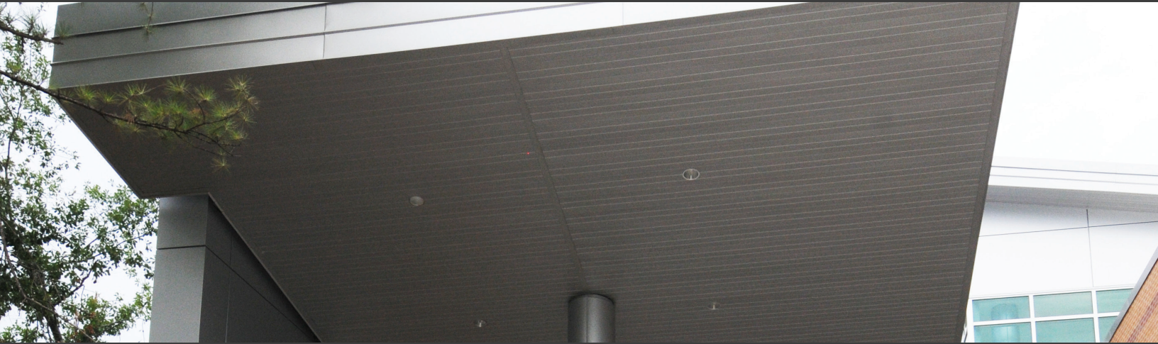
PROJECT: Texaco Service Station LOCATION: Beaumont, TX PANEL PROFILE: QwikLok™ COLOR: White
