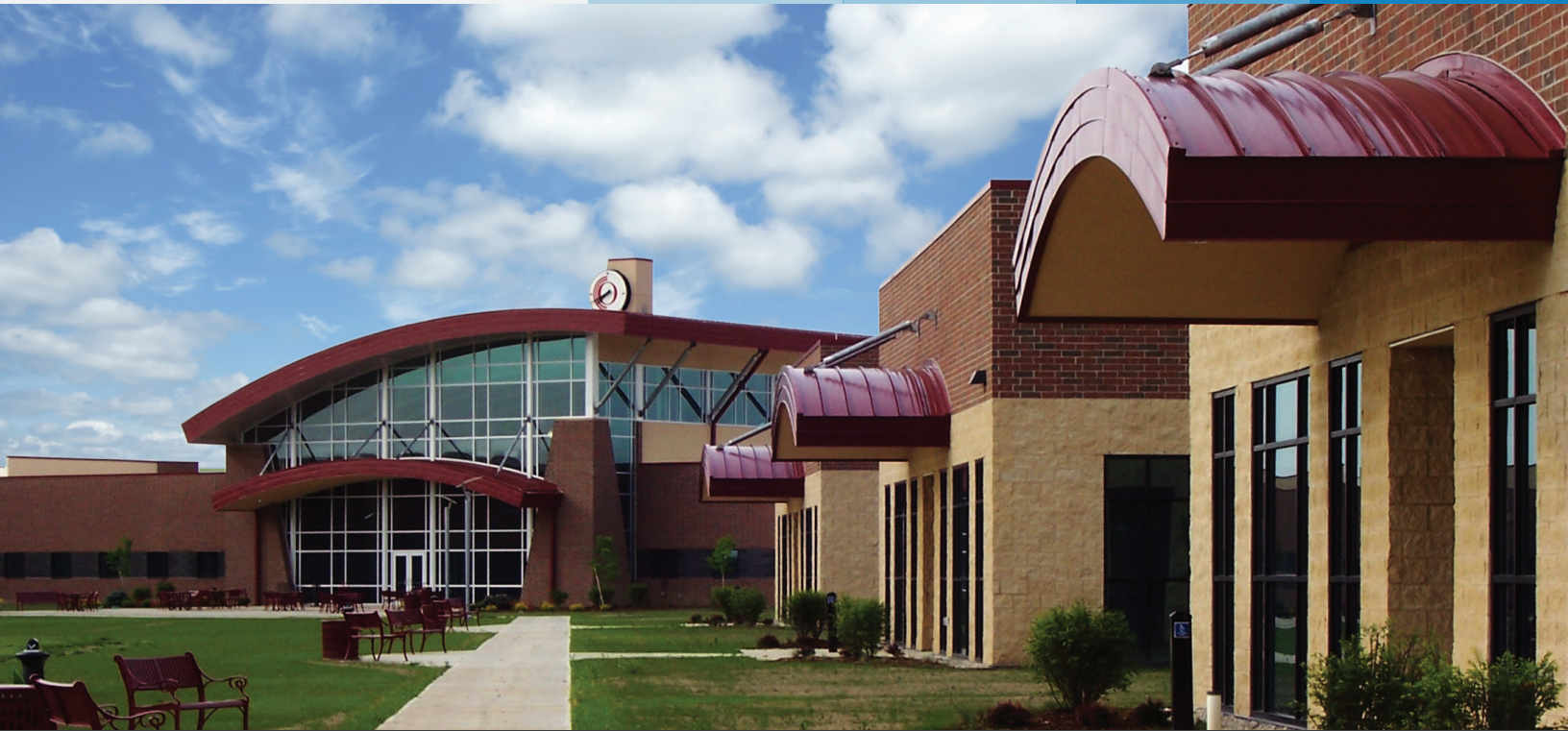
PROJECT: Owens Community College LOCATION: Fredericktown, OH PANEL PROFILE: Curved BattenLok® COLOR: Colonial Red
