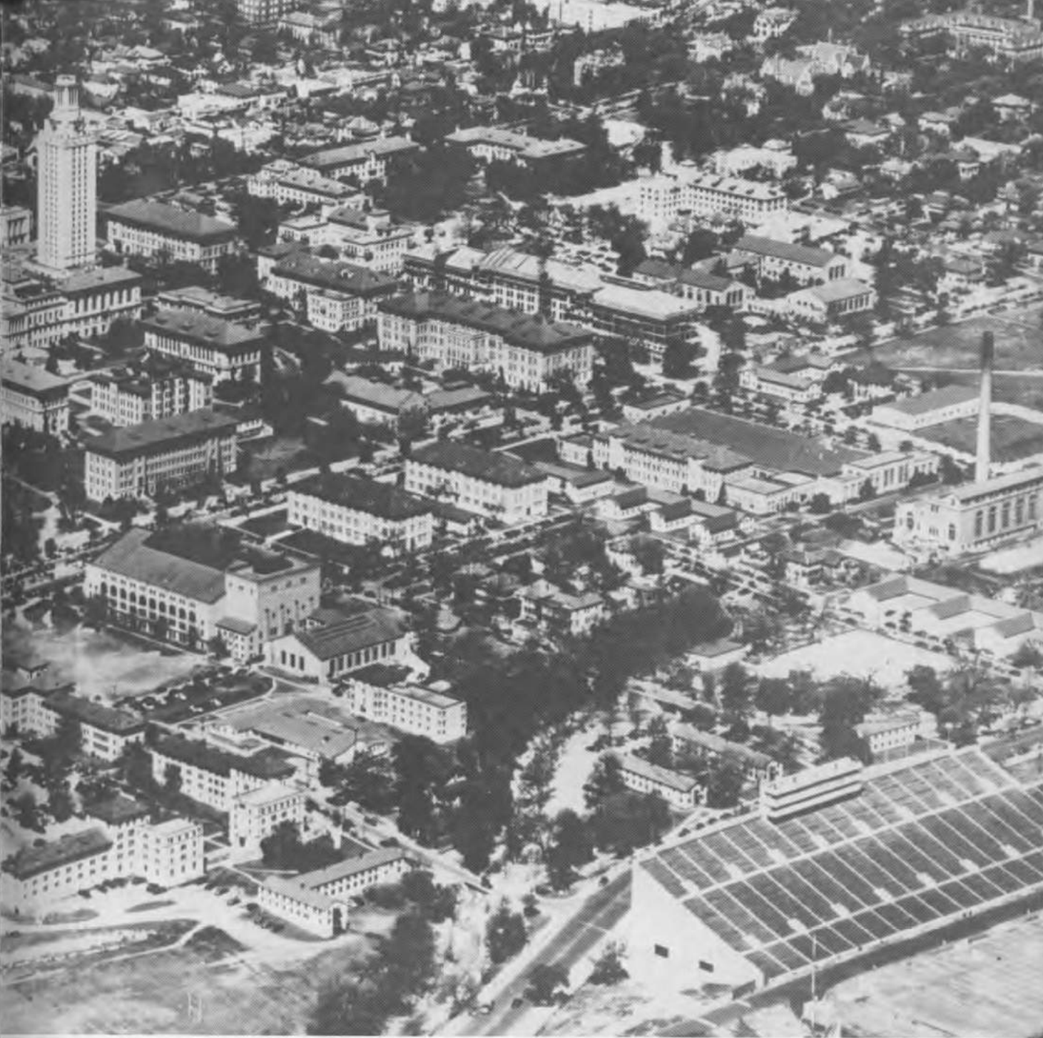
ESB is under construction.
