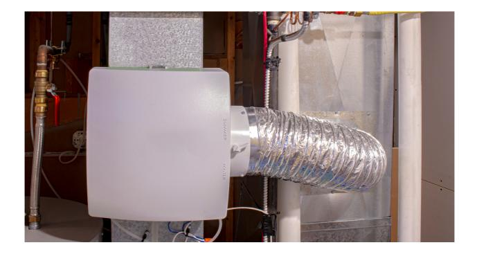
Use humidifiers with controls to reset the humidity level based on the outside air temperature. This combination will keep frost from forming as the chosen humidity level will be lowered while outside temperatures fall and be restored to normal during less severe weather.
