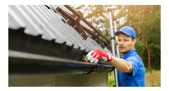
Clean gutters allow water to flow down easily from the roof and away from your home preventing damage to your foundation and ice buildup on your roof.
