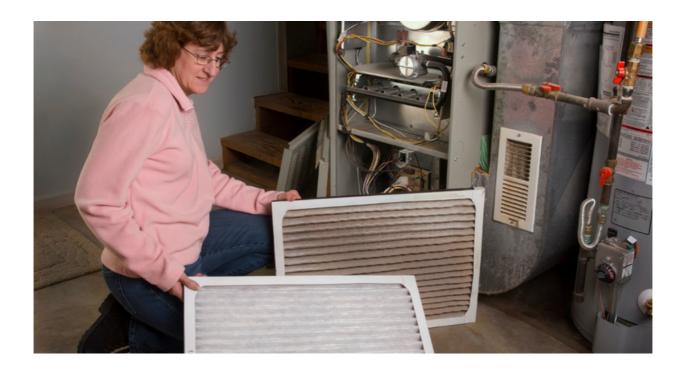
Replace the furnace filter every 3 months (more frequently if you have pets that shed fur) to ensure efficiency and keep dust particles from penetrating the clean, heated air. Inspect your furnace for leaks and test for carbon monoxide.
