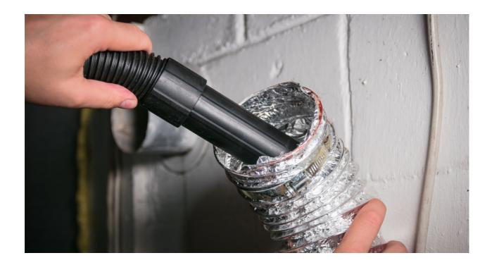
Dryer lint buildup in the duct behind the machine not only reduces the efficiency of your dryer but is also a fire hazard! It should, therefore, be inspected regularly.
