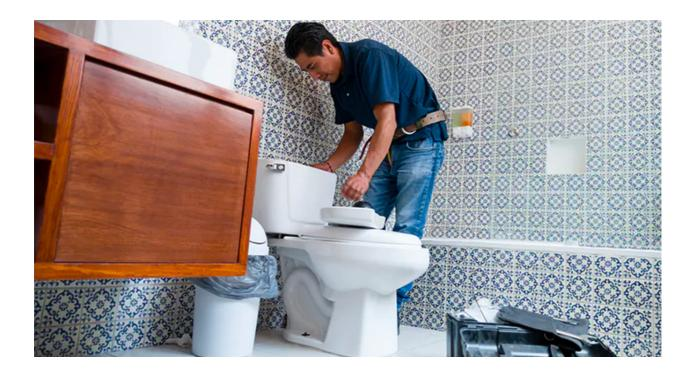
A leaky toilet can waste water and energy. Check for leaks by dropping some food colouring into your tank and then checking your bowl a short while later. If there is coloured water in the bowl then you have a leak and need maintenance.
