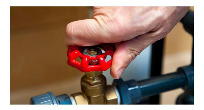
If a pipe becomes frozen, it can burst or leak, causing a flood in your basement. You need to know how to shut off the main water supply quickly so make sure you know where the main shut off valve is.
