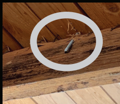
UNWANTED ROOF PENETRATIONS
