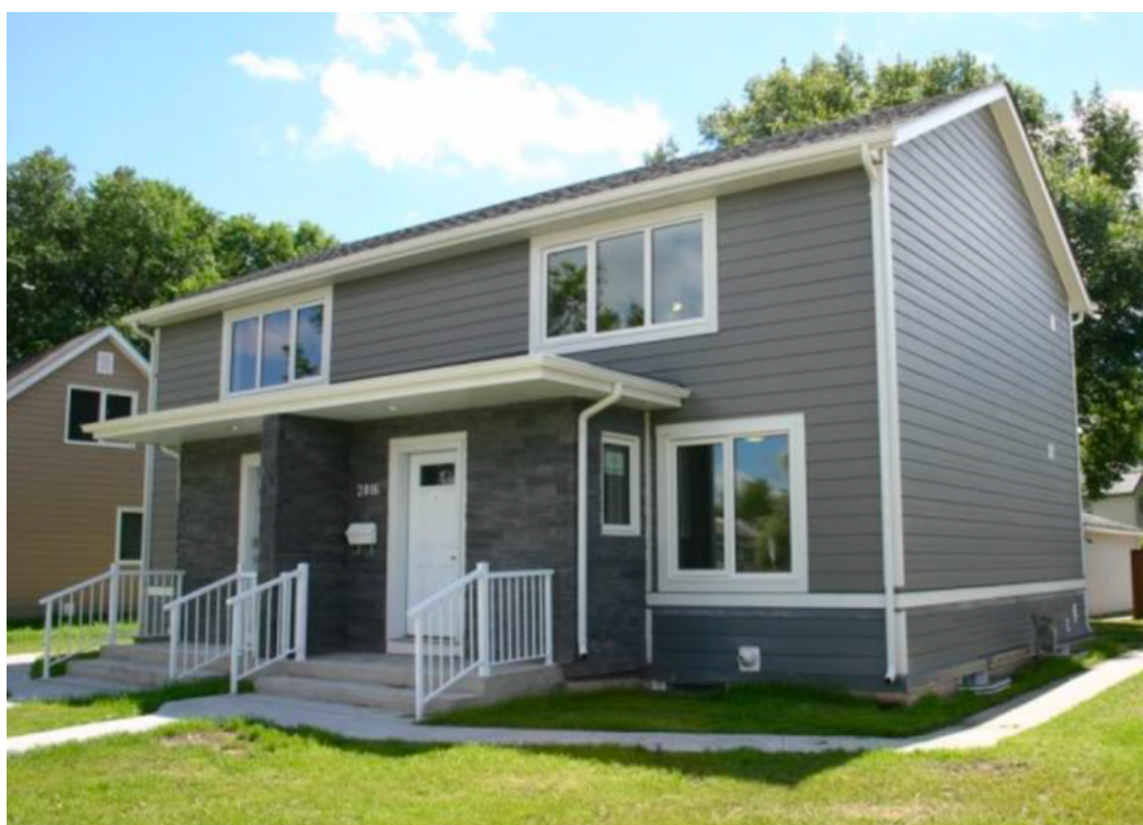
After: siding, trim, and other components installed. Proskiw Engineering Ltd., 2017.
