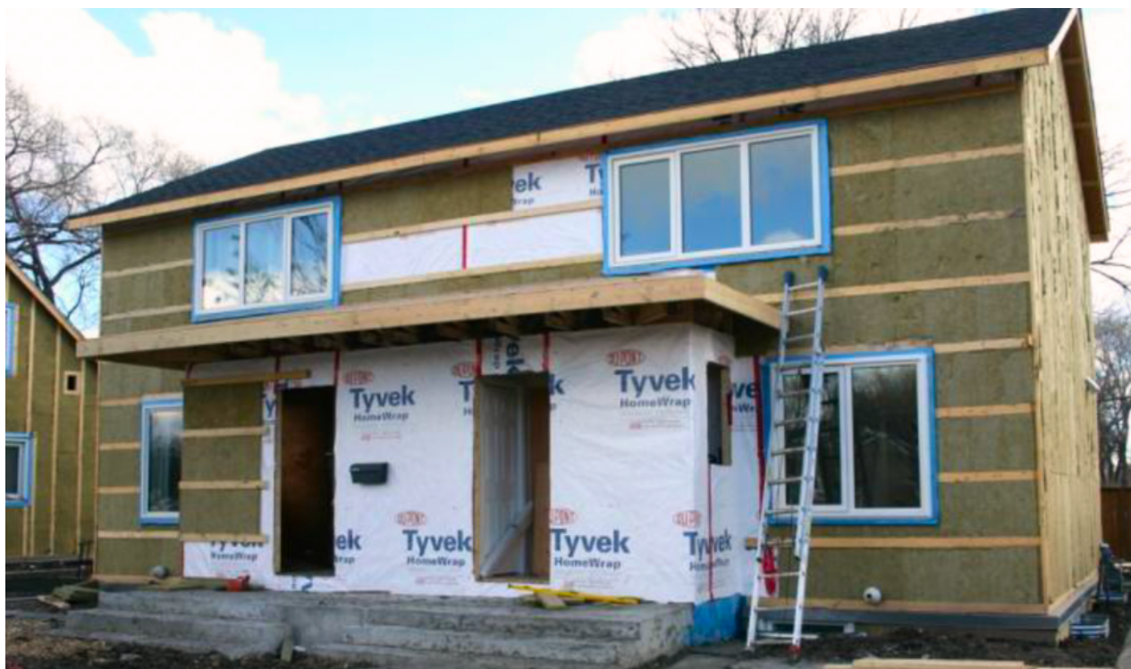
Before: mineral wool batts installed between horizontal strapping. Proskiw Engineering Ltd., 2017.
