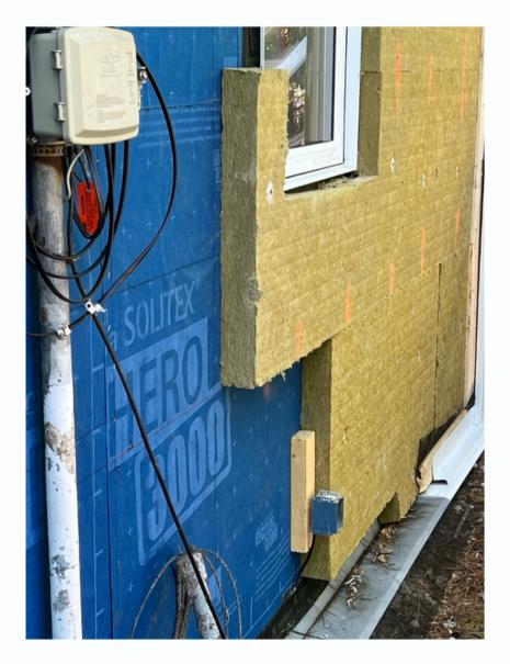
Once the existing cladding is removed, wall cavities can be easily filled or topped-up with insulation. Then, additional rigid or semi-rigid insulation can be applied over the existing sheathing prior to the new cladding being added. This will increase the wall thickness and significantly reduce heat loss. It also permits many of the air leakage pathways which exist through the walls to be sealed, further reducing heating and cooling costs.
