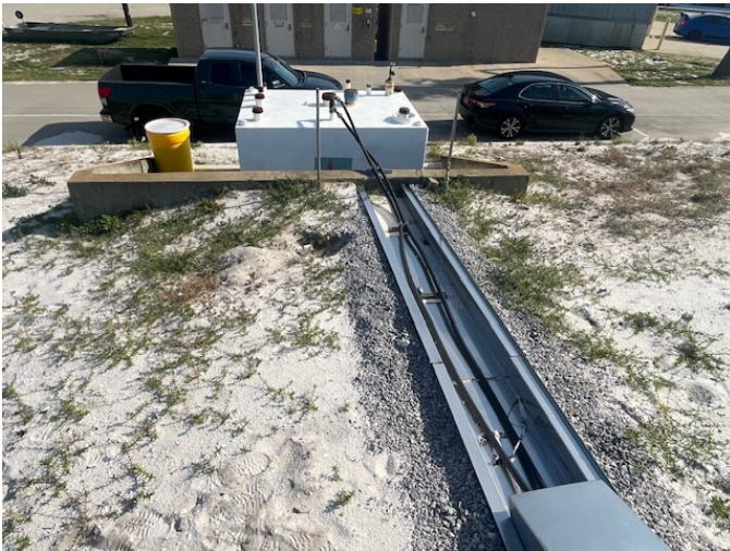
INVERT EXISTING TRENCH AS REQUIRED BY STATE, AND LOCATE AND SECURE EXISTING FUEL LINES TO INVERTED TRENCH
