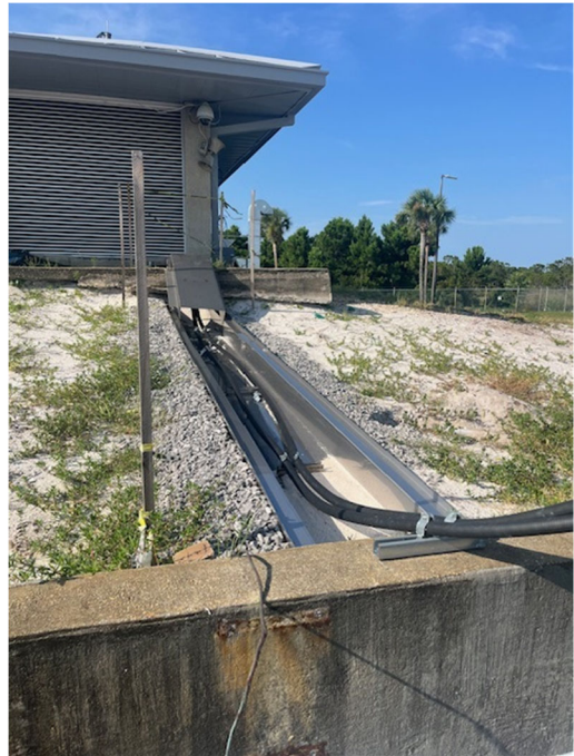
INVERT EXISTING TRENCH AS REQUIRED BY STATE, AND LOCATE AND SECURE EXISTING FUEL LINES TO INVERTED TRENCH
