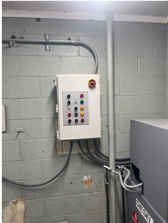
EXISTING DAYTANK CONTROLLER (LEFT) WITH 50 GALLON DAY TANK (RIGHT)
