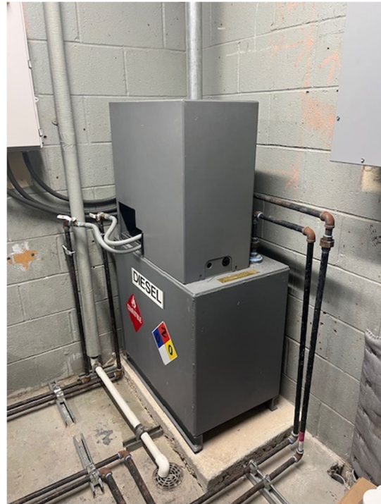
EXISTING DAYTANK CONTROLLER (LEFT) WITH 50 GALLON DAY TANK (RIGHT)
