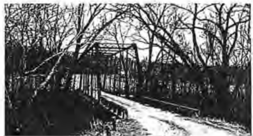
SULPHUR FORK BRIDGE 1888
