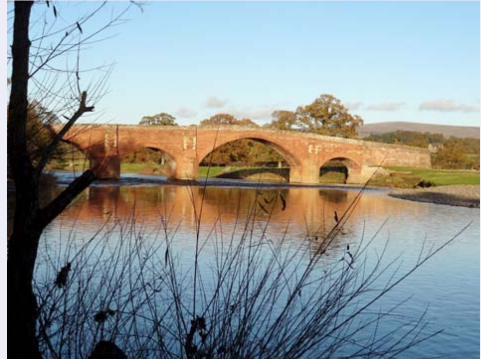
Lazonby Bridge, a classic River Eden bridge of local New Red Sandstone.
