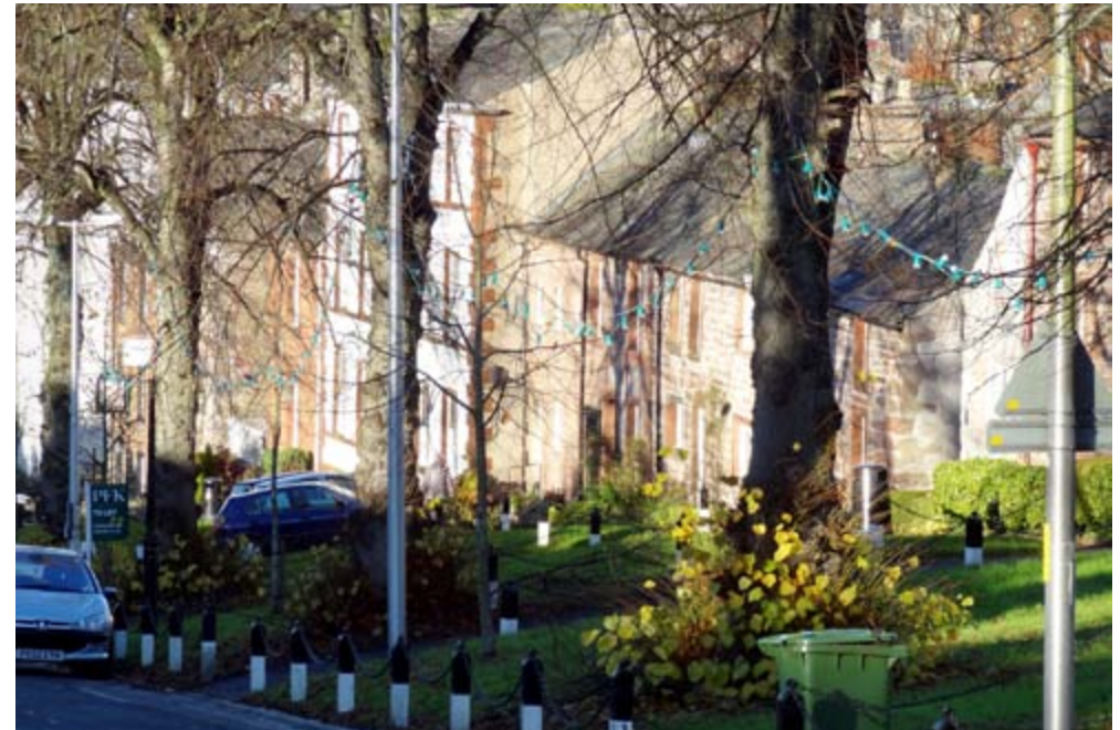
Boroughgate in Appleby-in-Westmorland, a small market town, once the county town of Westmorland, with a range of houses dating from the 15th-19th century and built in a mix of local vernacular materials.
