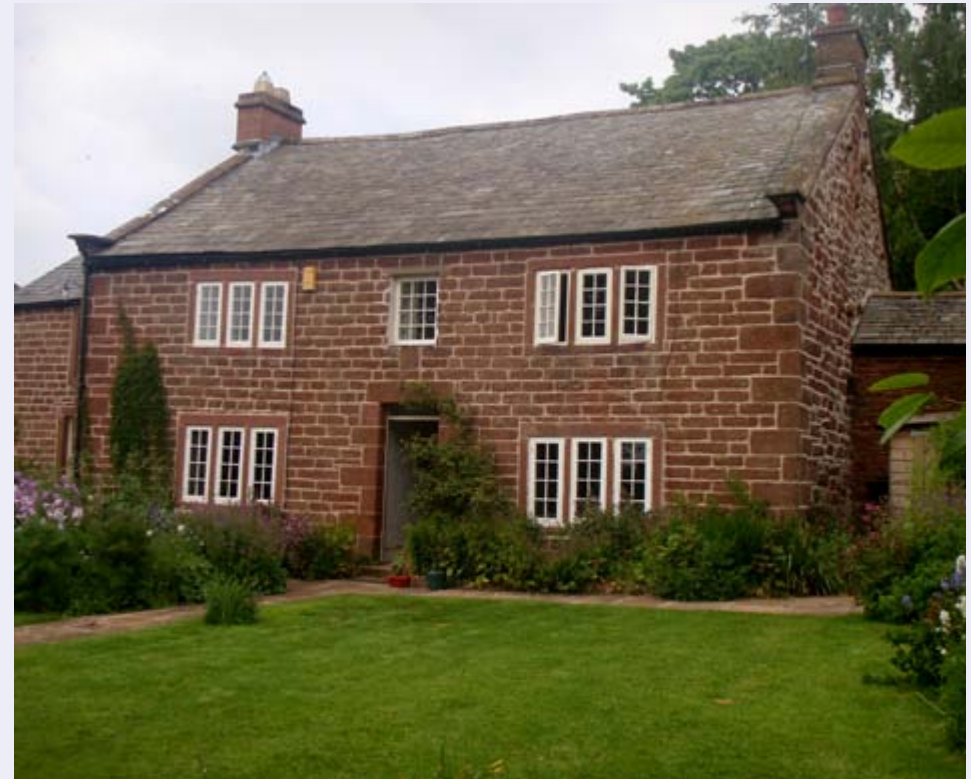
Typical Eden valley vernacular building style dating from the 18th Century: Westmorland slate roof and dressed New Red Sandstone walls, window and door surrounds, with a date stone over the front door.
