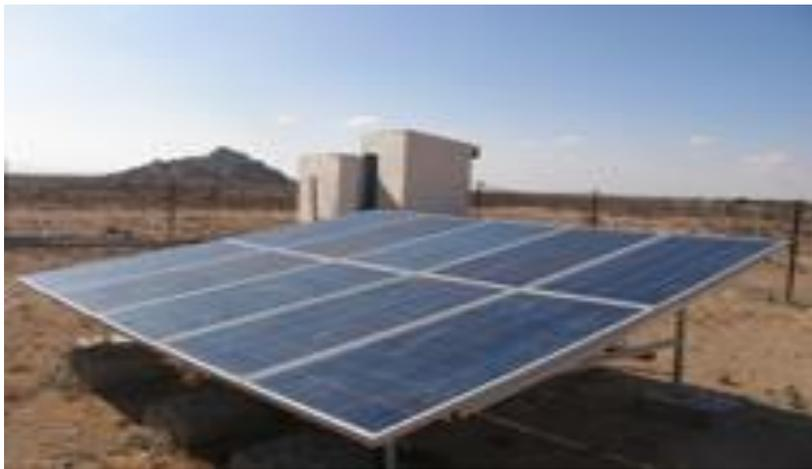
The solar panels installed on a high ground provide power to pump water distributed through a pipeline to the community, school and a health centre in Lasadacawo Village.
