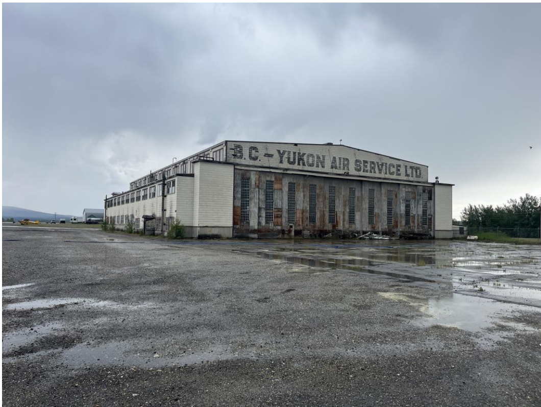
Abandoned Hangar in Watson Lake.
