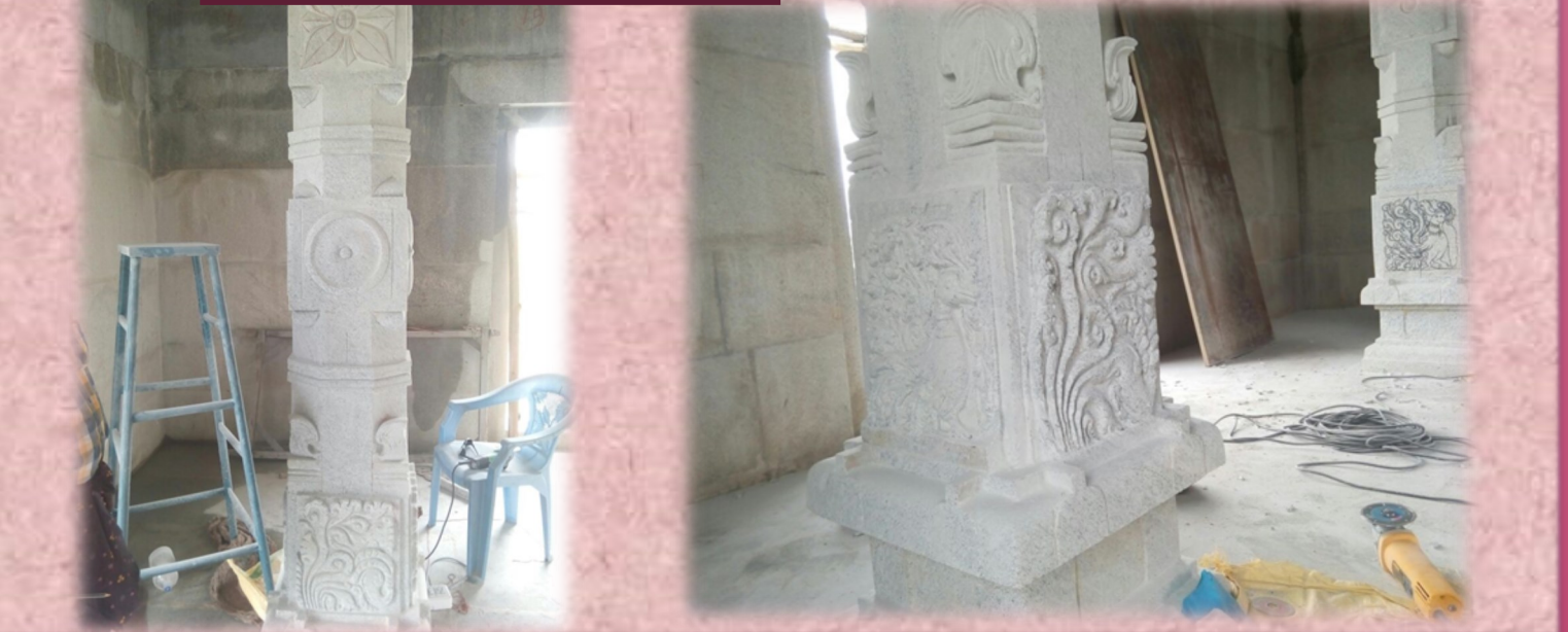
Intricate pillar carving work in progress
