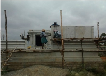
July 2014 Work on mandapam begins
