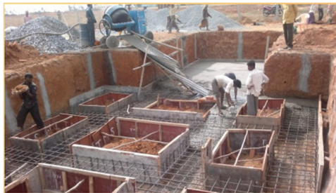
Dec 2011 Foundation Work for Temple
