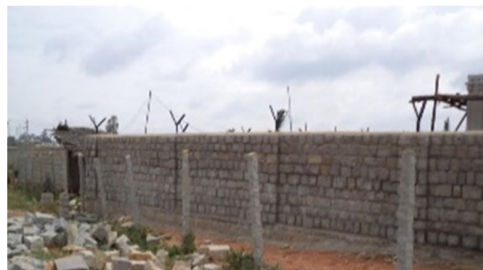
Aug 2013 Compound wall along the perimeter of the temple site built
