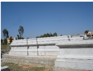
Jan 2013 Foundation for Garba Gruham complete
