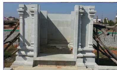
Nov 2013 Garba Gruham construction reaches half way stage
