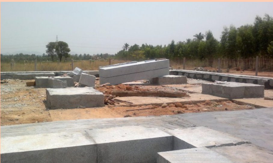
A few more stone blocks on the foundation.
