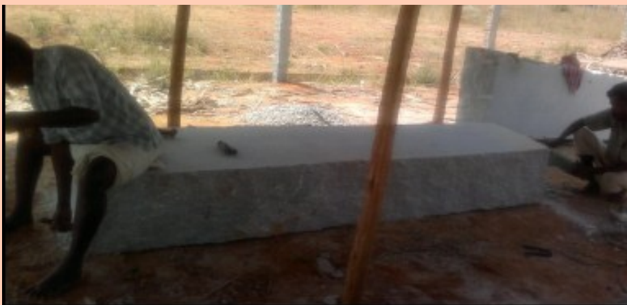
Carving work in progress inside the shelter.
