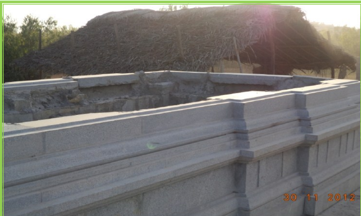
Stonework in progress, as Garbhagraham is being constructed
