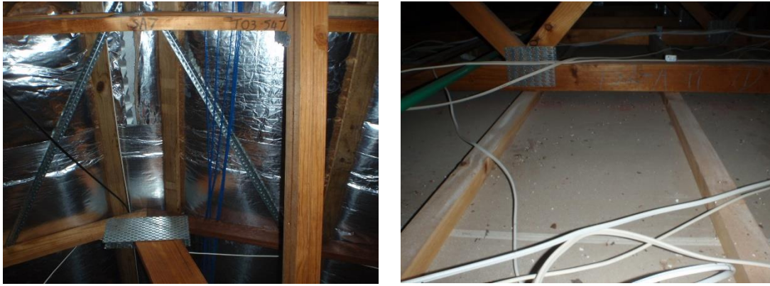
Figure 22: FNQ2 art centre building – roof with low thermal emissivity foil insulation and ceiling with no insulation
