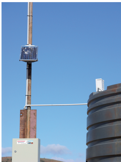
Figure 12: Examples of telemetry systems used to remotely monitor water points
