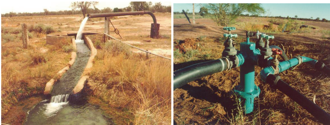
Figure 1: Open drain and reticulated watering systems
