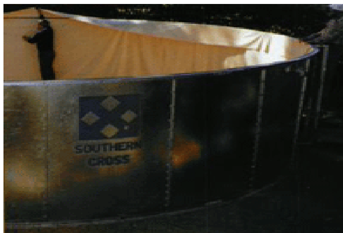
Figure 15: Example of a plastic lined modular steel tank
