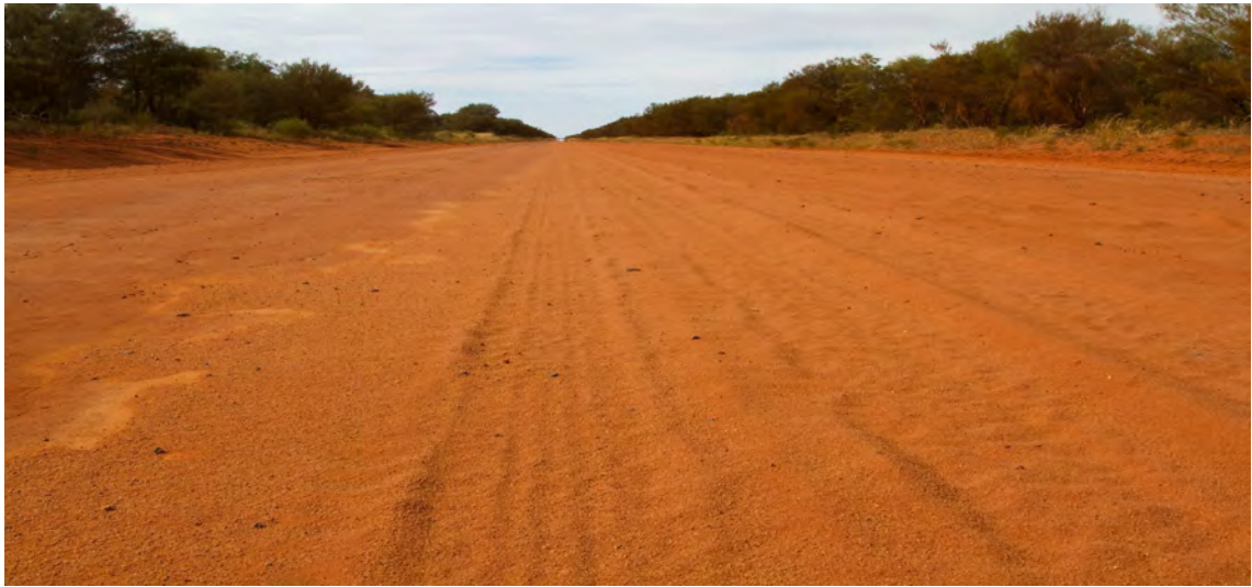
Photograph 4: The Tanami Highway is subject to major corrugations and flooding, May 2014 (Photograph Kim Petersen).
