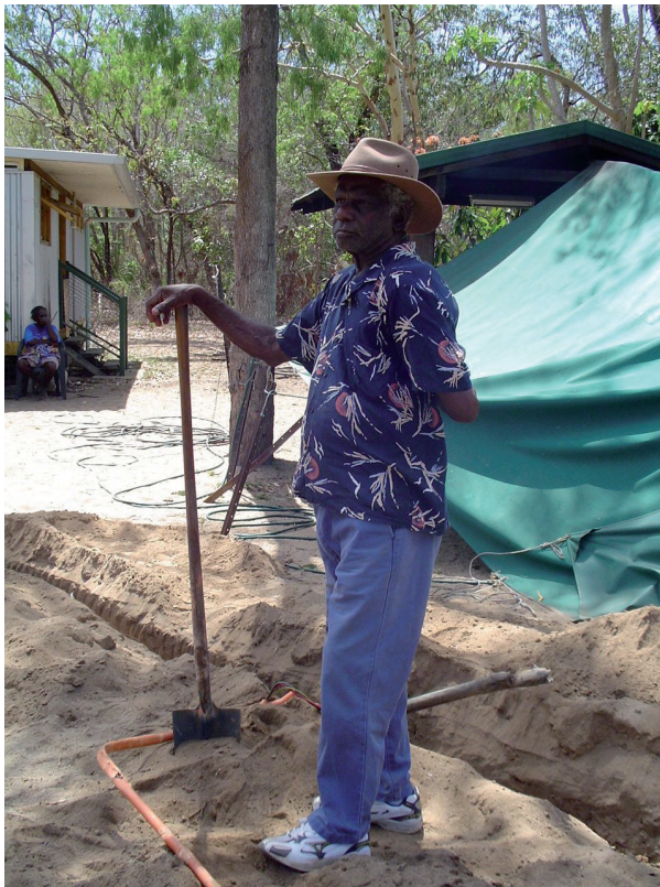
Figure 12: Sunlight Bassini repairs the water pipes at Port Stewart
