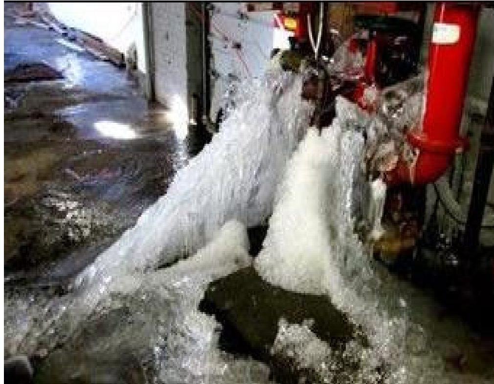
Frozen Fire Protection in unheated stair well
