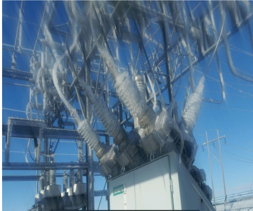
Frozen insulators can short equipment
