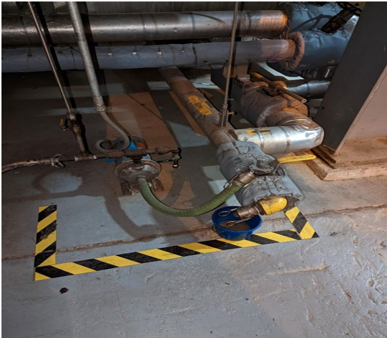
Offline boiler recirculation pump
