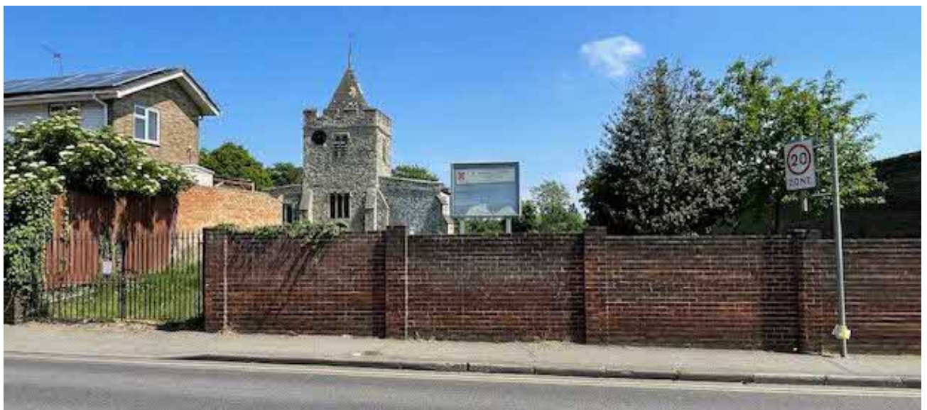
Figure 5. Churchyard Entrance Gate - Vehicular Access (Ship Lane)
