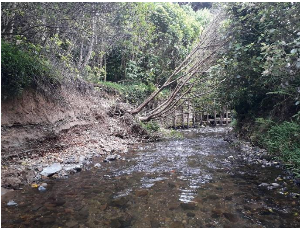
Plate 17: Transect 024/02 – Eroded stream bank and degrading erosion protection structure. Established riparian vegetation. Tradescantia present.
