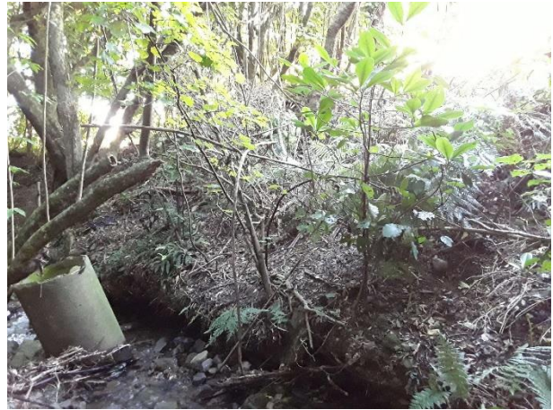
Plate 28: Transect 027/03 – Moderate density riparian vegetation. Concrete structure present within stream channel.
