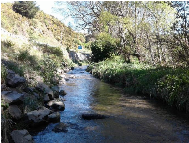
Plate 15: Transect 024/00 – Stream parallel to Middleton Road, stream armouring present on the true right.
