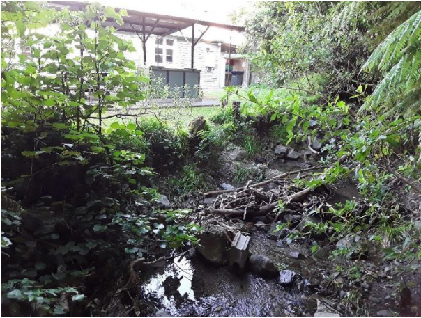
Plate 27: Transect 027/02 – Stream channel next to Camp Elsdon. Foreign materials within stream channel.
