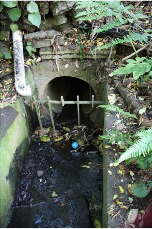
Grill. Debris arrester installed by Makara County Council about 8 inches in front of the stormwater pipes.
