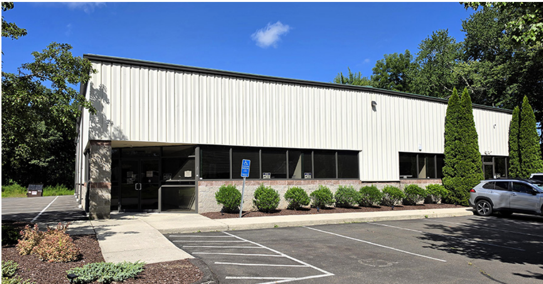
Figure 4. Microscreen's new 8,000-sq.-ft. SMT solder stencil manufacturing facility in Oxford, CT.
