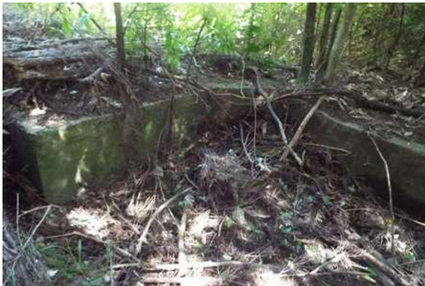
Sump in Centre of Site
