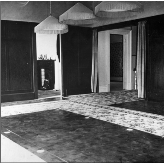
Billiard room and entrance to upstairs hallway
