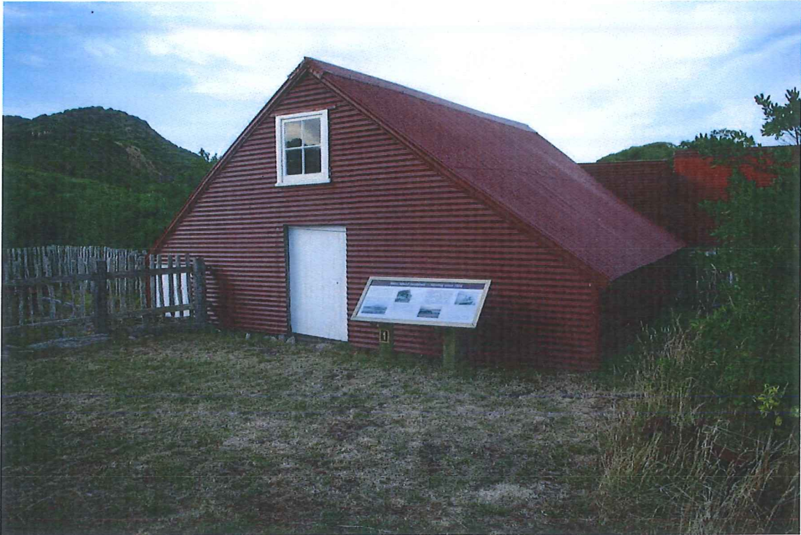
Woolshed building viewed from the southwest (Dodd, 07.03.2019)
