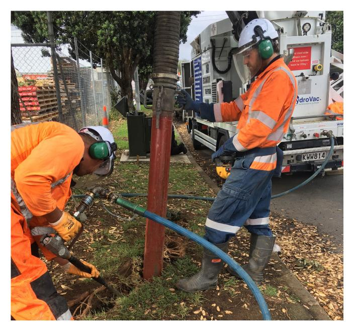
HydroVac's Dry X trucks offer an extensive reach of 150m so they also work well in smaller, hard-to-reach areas. The trucks have been configured for reduced noise pollution, helpful for work in suburban areas, and are fitted with an unique filtration system that prevents them from emitting dust into the atmosphere when they operate.
