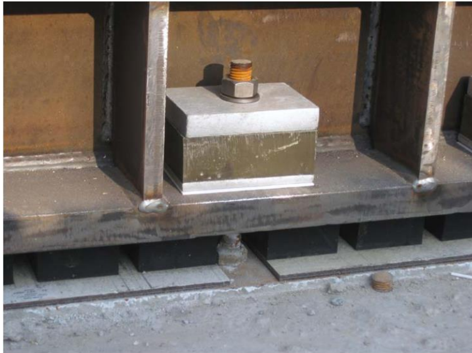
Figure 1. An example of an elastic bearing in a building foundation (Source CDM Group)
