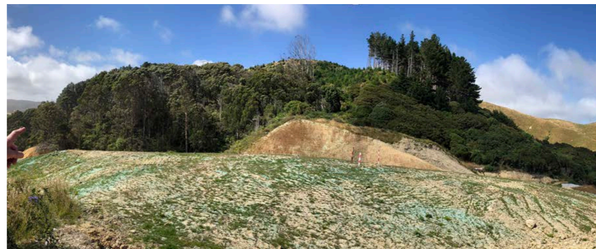
looking south over Lot 6 from north side of Link Road
