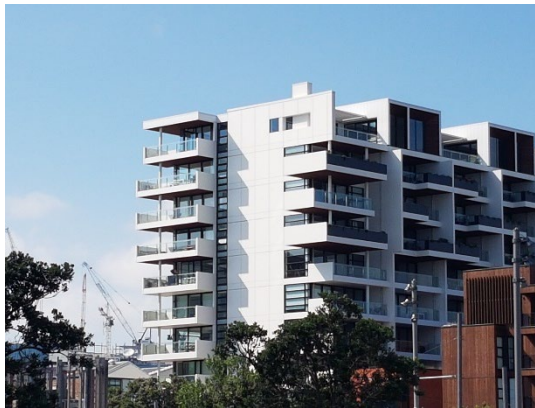
Visual bulk of building modulated with variation in roofline and façade alignment, and projecting and recessed balconies.
