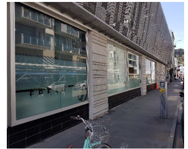
This inner-city supermarket presents display windows to the street, and conceals its upper level carpark with an architectural screen
