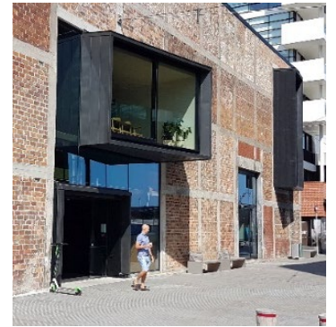
Expression of building entry
