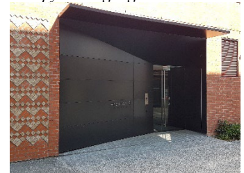
Apartment entrance from a lane signalled with setback, canopy and contrasting colours and materials
