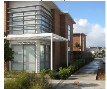
Privacy at a street corner achieved with a shallow setback, louvres at high level and internal window treatments
