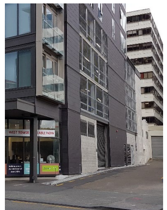
Servicing located under and behind the building in combination with carparking screened by a veneer of apartments fronting the street
