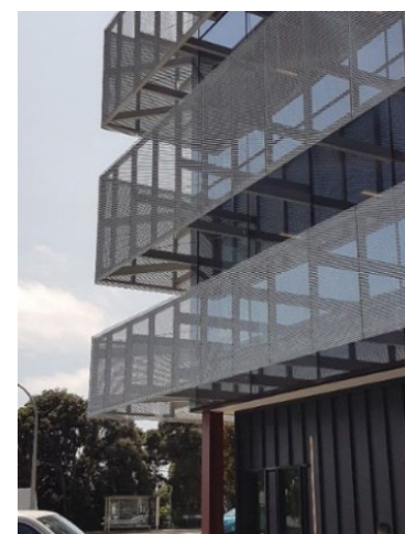
Shading devices articulate the façade of this large format building
