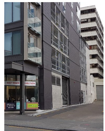
Servicing located under and behind the building in combination with carparking screened by a veneer of apartments fronting the street
