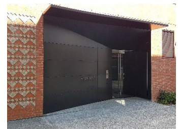
Apartment entrance from a lane signalled with setback, canopy and contrasting colours and materials
