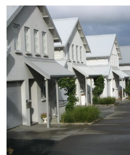
Entry porches and windows to habitable rooms fronting to the street. Single garage doors are located at the frontage but are not prominent in views along the street
