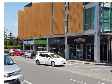
A long frontage articulated with multiple shopfronts at ground
