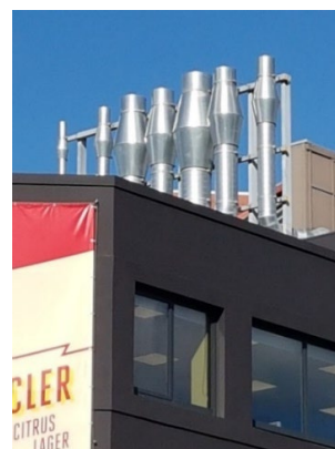
Flues grouped as a feature on a rooftop
