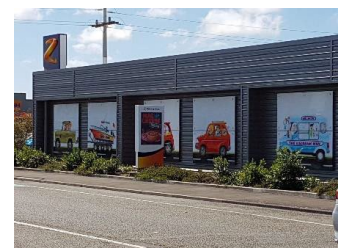
Façade treatment to the otherwise blank back of a service station kiosk at the street edge, utilising façade variation and graphics that relate to the service station function.
