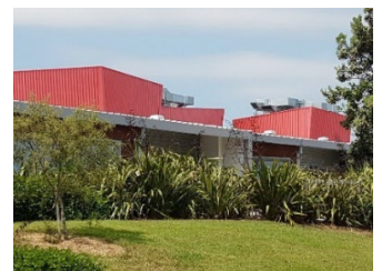
Plant enclosures as sculptural forms lend visual interest to a large floor plate roof form
