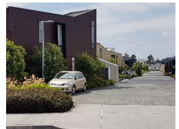
Shared surface rear access lanes which incorporate planting and subtle variation in paving and are overlooked from the houses served
