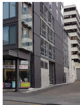
Servicing located under and behind the building in combination with carparking screened by a veneer of apartments fronting the street
