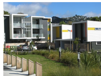
Shared outdoor area at the centre of a large development. Units front the spaces which in this case provide for public access through.
