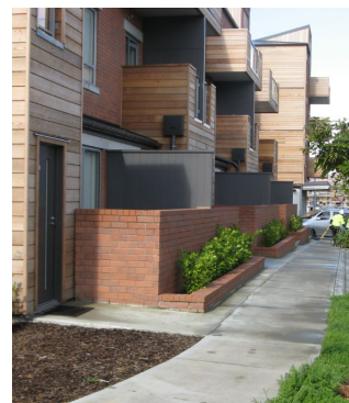
Wing walls between units allow small outdoor living areas at the street edge a reasonable degree of privacy.
