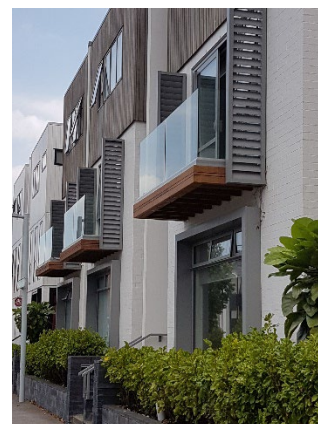
Balconies opening out to the street edge from upper level living room, and ground floor privacy achieved with window setbacks and edge planting
