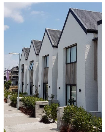
Planting and low fences give suitable privacy and present a positive edge to the street
