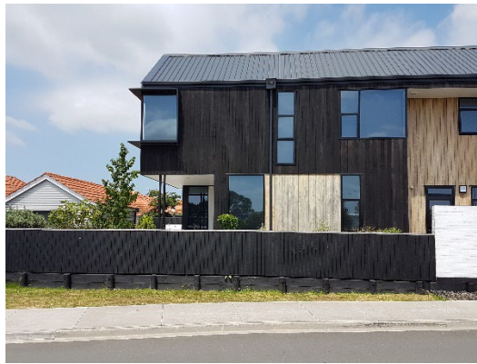
Visual interest achieved on large walls with variation in materials within a carefully proportioned composition
