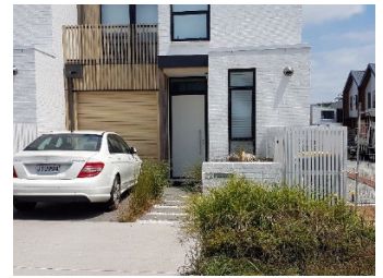
Garage in a terraced housing development is unobtrusively located next to the front door and well back from the street edge
