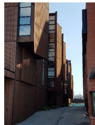
Apartment windows looking along a lane and orientated to avoid short range views into townhouses across the lane
