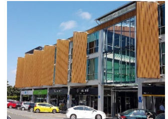
Subdivision and modelling of form and façade to reduce the apparent visual bulk of a building
