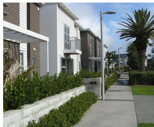
Projection of window bays, stepping of forms and gaps between units contribute visual interest to a terraced development. These images also show the value of frontage planting in adding to the visual richness and street appeal of the units.
