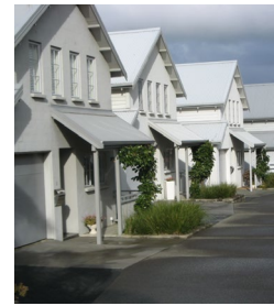
Entry porches and windows to habitable rooms fronting to the street. Single garage doors are located at the frontage but are not prominent in views along the street
