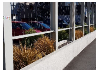
Landscape treatment to the street edge of a carpark including a frame, low wall and planting
