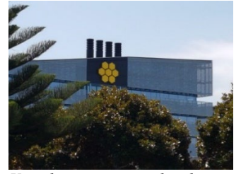
Visual interest created with change to roof plane and visual expression of services on the roof-top
