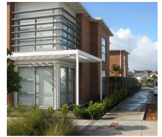
Privacy at a street corner achieved with a shallow setback, louvres at high level and internal window treatments
