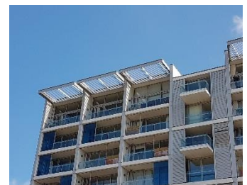
Recessed balconies with sliding screens provide for sunshading and privacy while adding further visual richness to the façade
