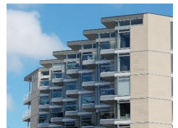
Windows and balconies on a high-rise apartment block are oriented to optimize views as well as sun and privacy
