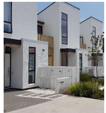
Bin storage discreetly located and screened readily accessible from the front door and close to the street edge in this townhouse development
