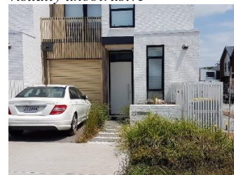
Garage in a terraced housing development is unobtrusively located next to the front door and well back from the street edge
