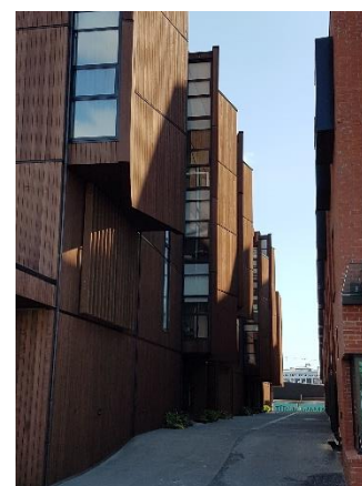
Apartment windows looking along a lane and orientated to avoid short range views into townhouses across the lane
