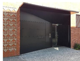
Apartment entrance from a lane signalled with setback, canopy and contrasting colours and materials
