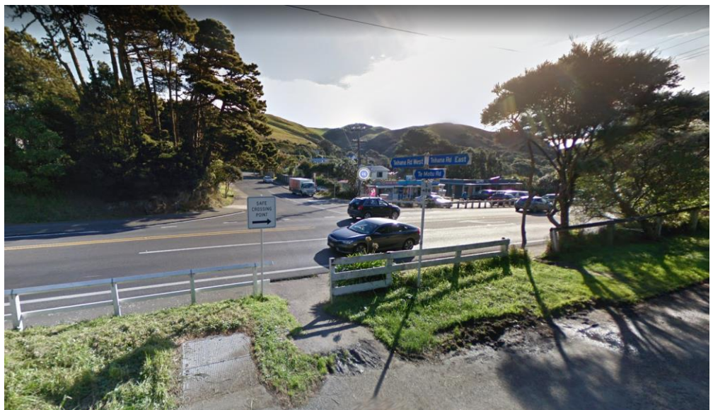
Figure 3: View in the direction of the railway station across SH49 to Teihana Road East. The sign in the foreground reads: 'Safe Crossing Point' with arrow pointing to the crossing some 50m to the north as identified on Figure 2.
