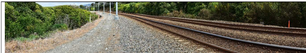
Figure 14. Panaroma showing culvert physical location.
