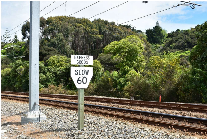
Figure 12. Speed restriction approaching Plimmerton station.
