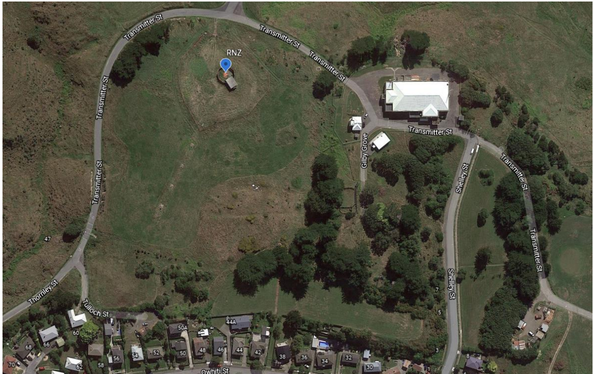
Figure 1: Location of RNZ’s Porirua transmitter site.
