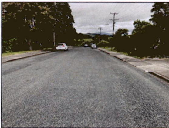
Photo 6 View to S along Rawhiti Road close to road-end (November 2018)
