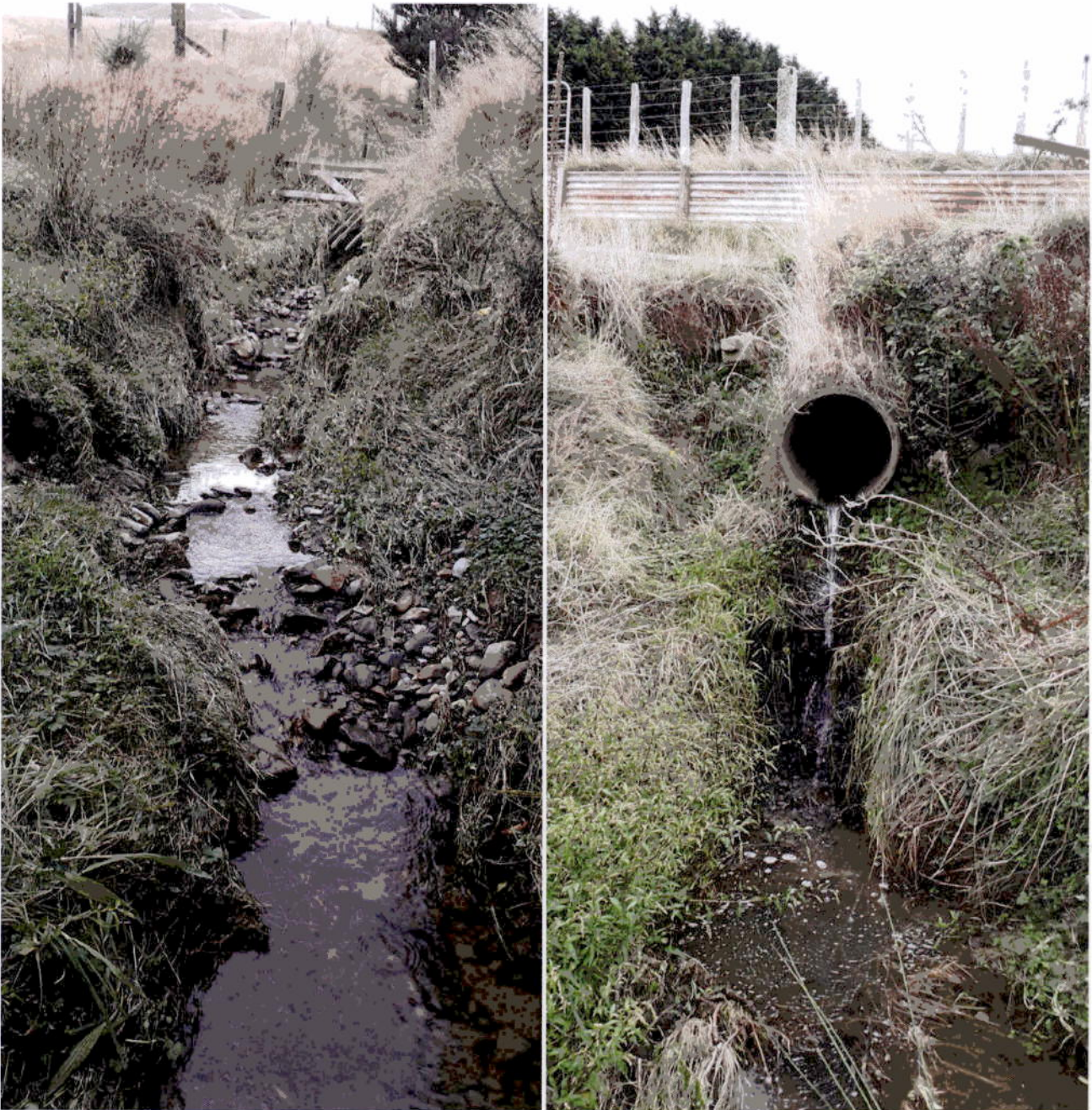
Figure 1: (left) The lower reach of the stream onsite (right) the perched culvert beneath the farm track.
