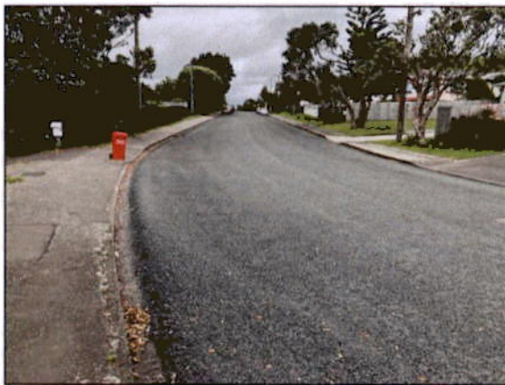
Photo 5 View to S along Rawhiti Road (November 2018)
