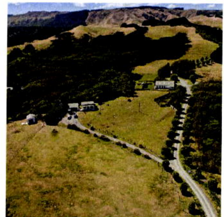
Figure 14: The driveway providing access to buildings on the site.
