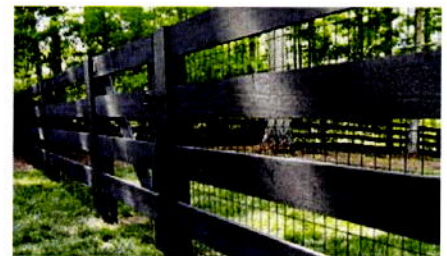
Figure 41: Black post and rail fencing with black wire mesh between green fingers and properties.
