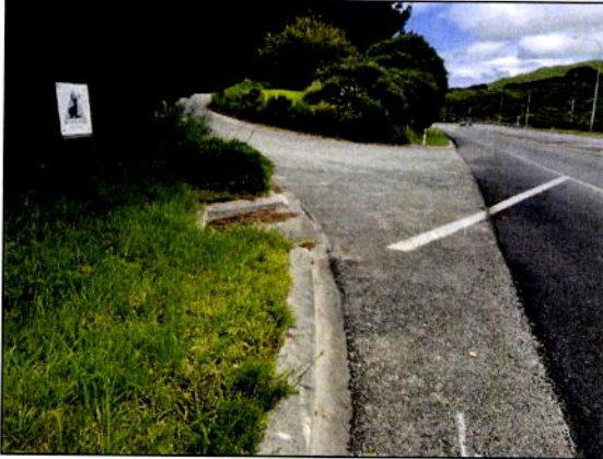
Photo 4 View to SW across Mt Welcome Station access (November 2018)
