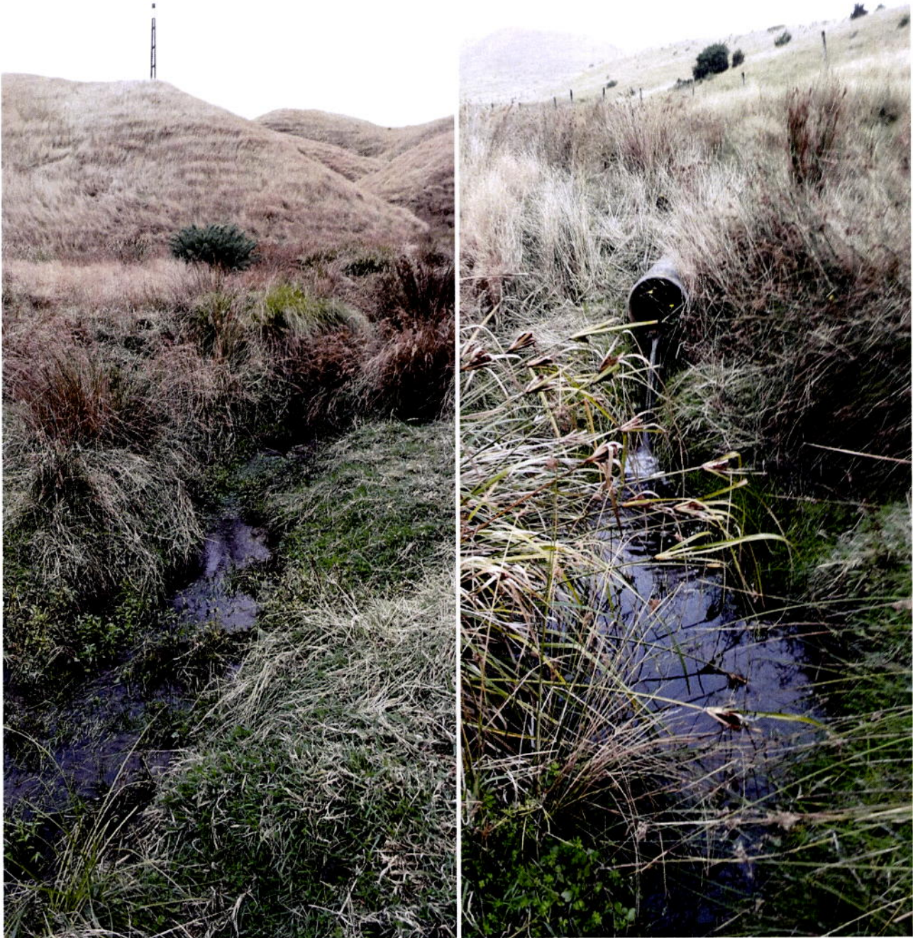
Figure 1: (upper) The lower reach of the stream at the southwestern boundary of the site (lower) a perched culvert beneath a farm track in the same stream.
