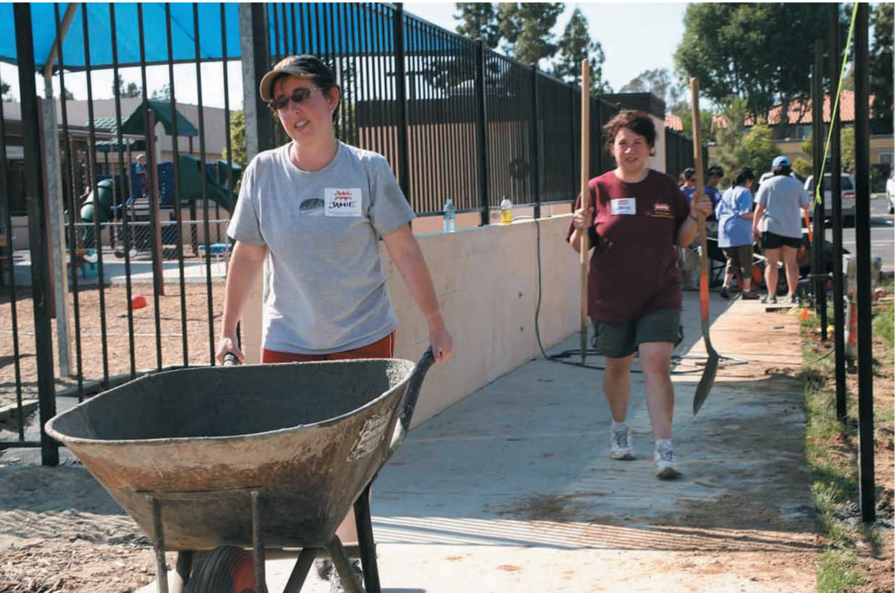
MedImmune's Jamie Lacey, Senior Director, Media and Public Relations, pushes a wheelbarrow full of concrete in preparation for building the playground in Escondido, Calif.
