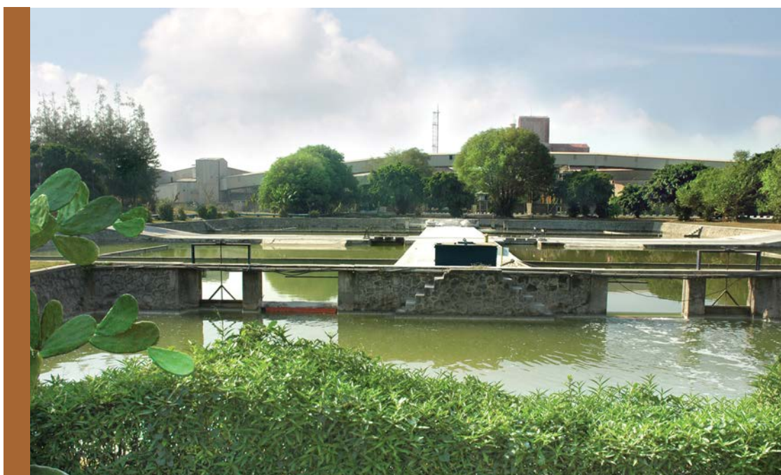
Unit Pengolahan Limbah Cair / Waste Water Effluent Treatment Unit
