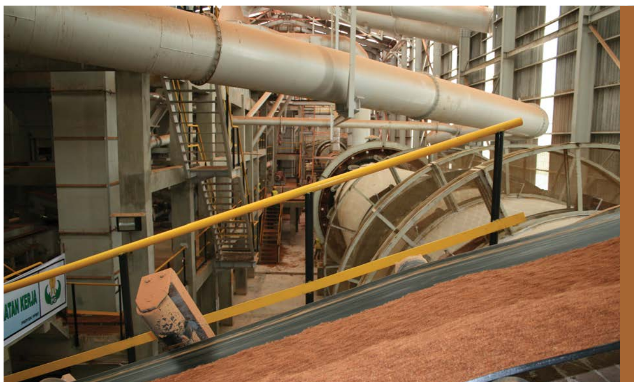
Pabrik NPK III & IV / NPK Plants III & IV
