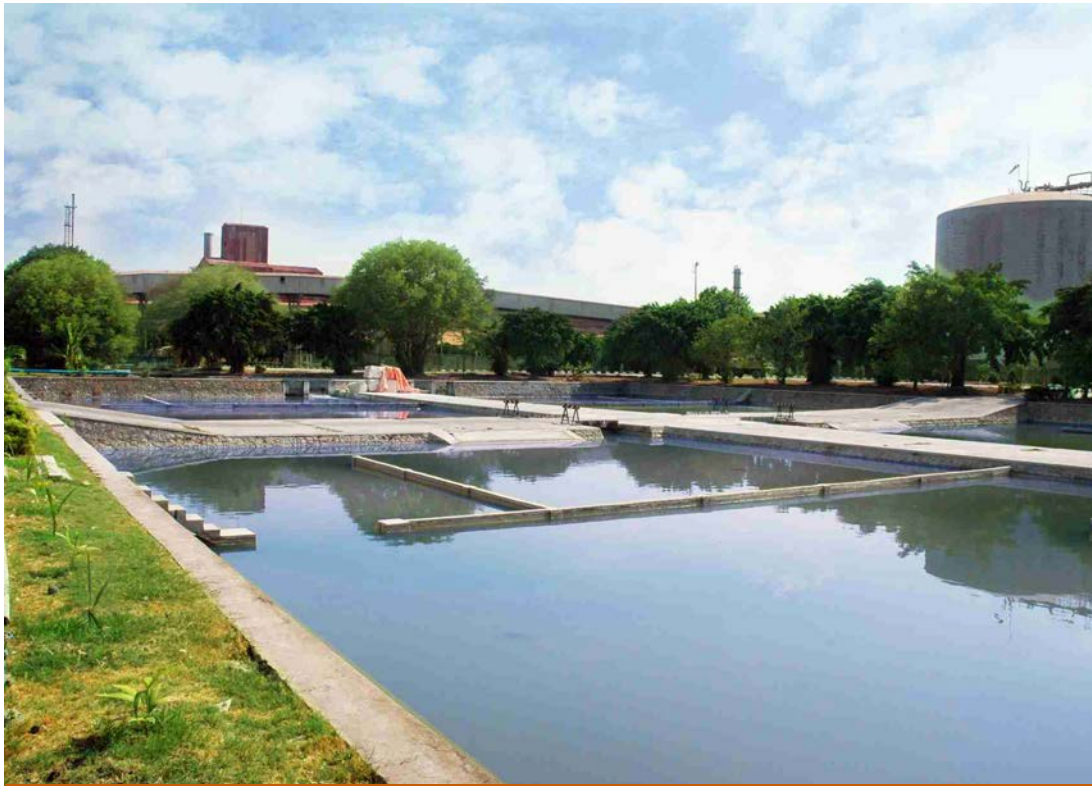
Unit pengolahan limbah cair PT Petrokimia Gresik Liquid waste treatment unit of PT Petrokimia Gresik
