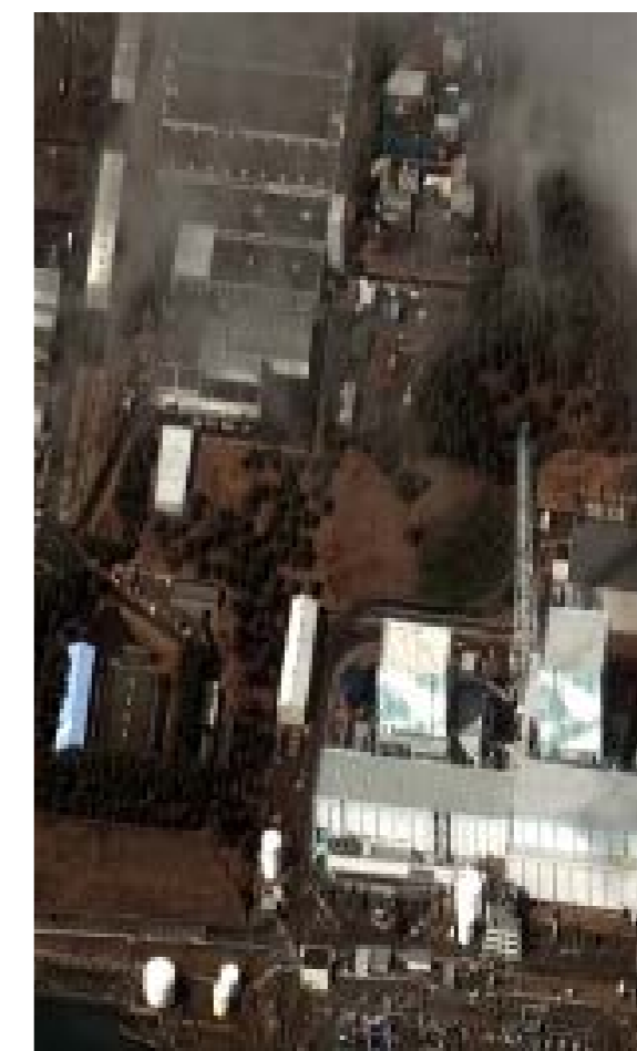
Fukushima I Nuclear Power Plant Damage
